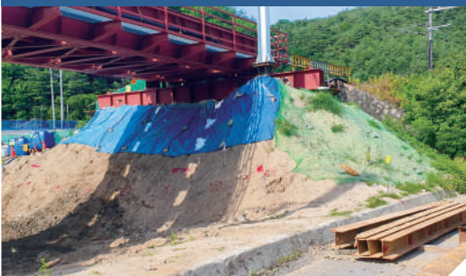
HEAD ROOM CONSTRUCTION
