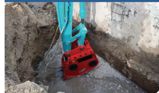
UNDER WATER OPERATION
