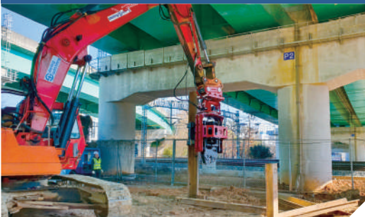
HEAD ROOM CONSTRUCTION
